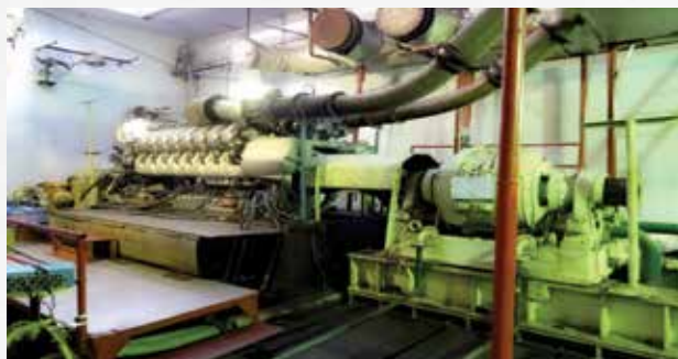
Engine Undergoing Full Power Trials at Test Bed No 1
