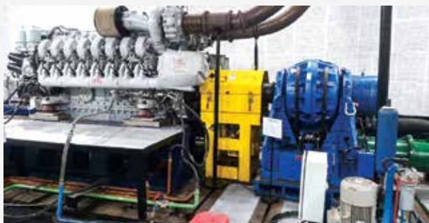
Full Trials of Engine at Newly Inducted Test Bed No 2
